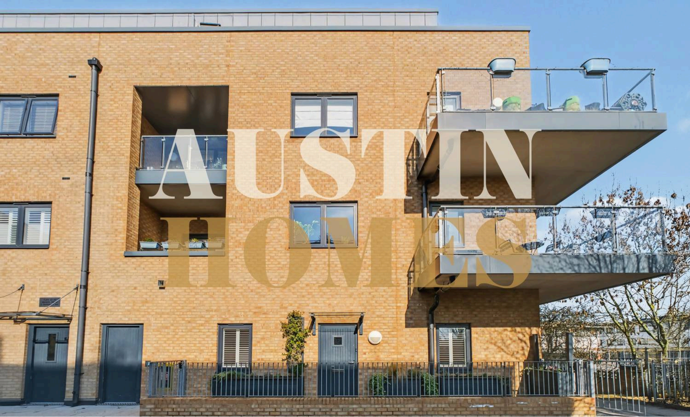
Arundel House, 3 Thornbury Way London
